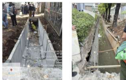
Figure 1. Elevation Measurement on One of The Channel Segments
